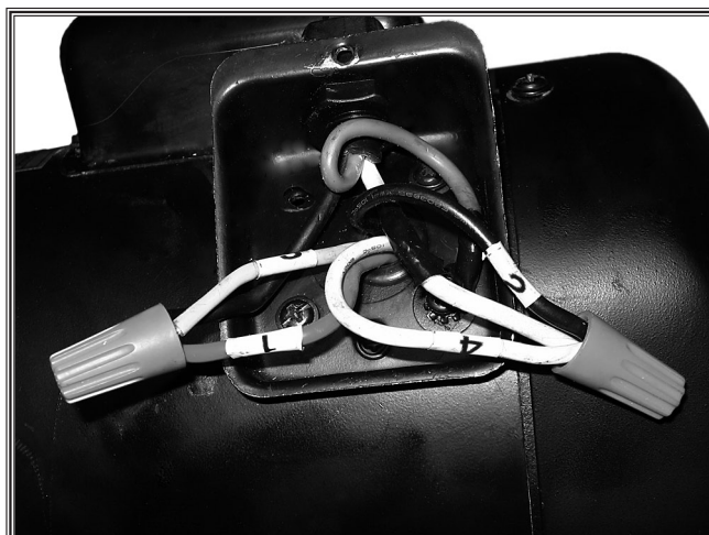
Figure 45. 110V motor wiring.
