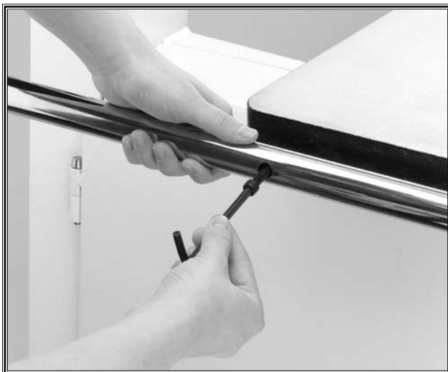
Figure 22. Securing rail with cap screw.
